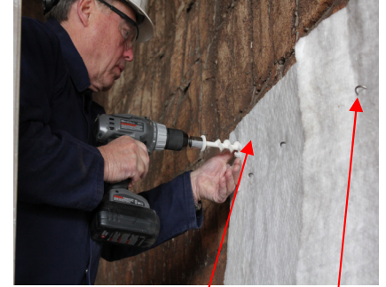
Normal Fiber Blanket Spacing (Temporary Retaining Clip)
