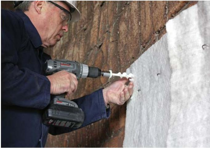
**Fig. 3. Drilling bolt into a lining**
