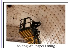
Hi-Alumina Retention System STELBOLT<sup>TM</sup> was designed to both repair and compliment existing light weight insulating furnace linings.
