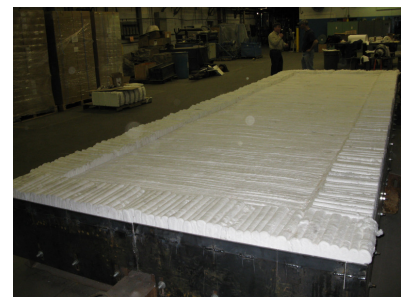
Completed MAFTEC® Installation
